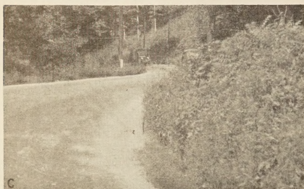
WEEDS MAY BECOME A MENACE TO TRAFFIC: A, BY REDUCING THE EFFECTIVENESS OF GUARDRAIL; B, BY CONCEALING MARKERS AND OBSTRUCTIONS OUTSIDE THE TRAVELED WAY; AND C, BY SHORTENING SIGHT DISTANCES AT CURVES.
